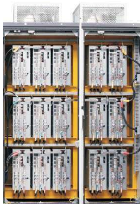
Fig 3.7 Layout in the power unit cabinet
